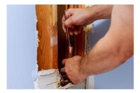
**1. Locate the Source.** To the extent possible, determine where the water is coming from. A leak may be inside walls, in sink plumbing lines, toilets, washers, angle stops, or from a hot water heater. If you're unable to readily locate the source, determine the most likely culprit. Is it near a window? A ceiling leak could be from the roof or an upper unit.
